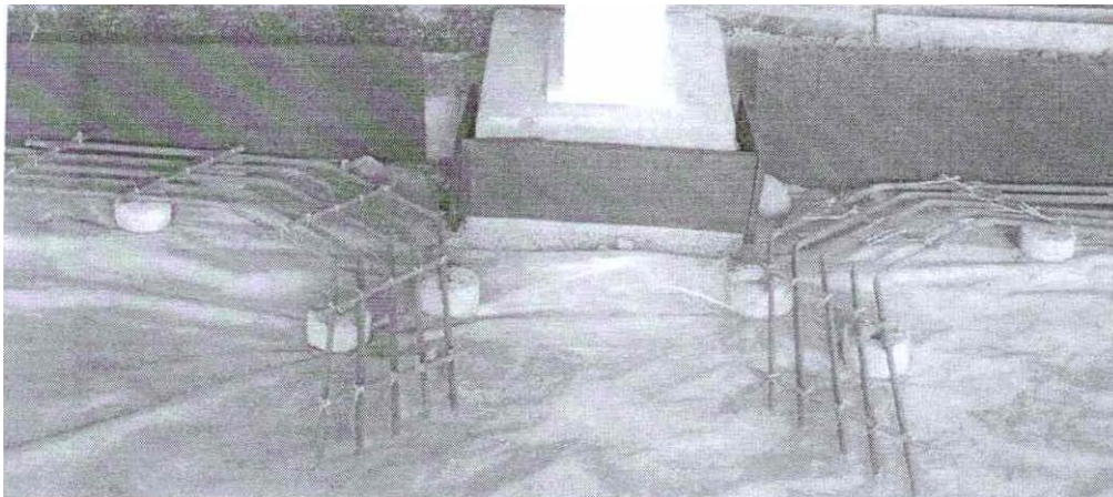
One Stage Construction: Column Isolation & Auxiliary Reinforcement.
